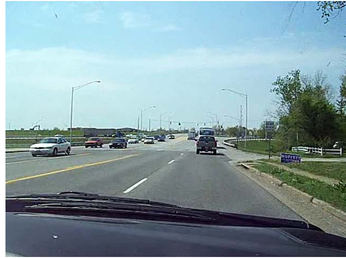
KY 54 Approaching US 60 Interchange
