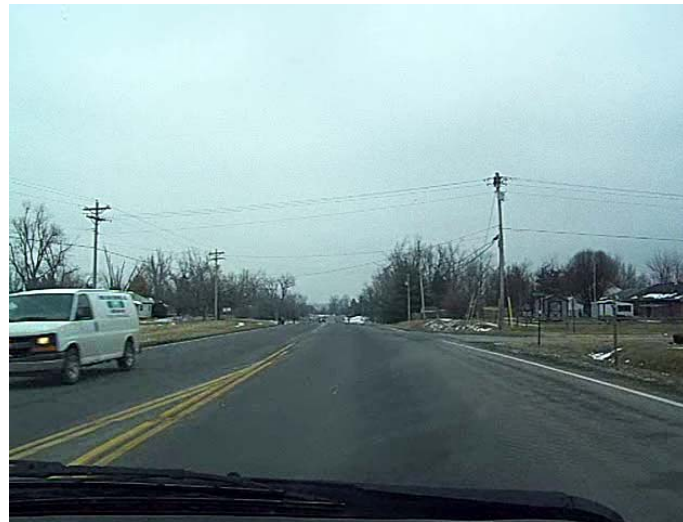
KY 54/Waterwheel Way Intersection
