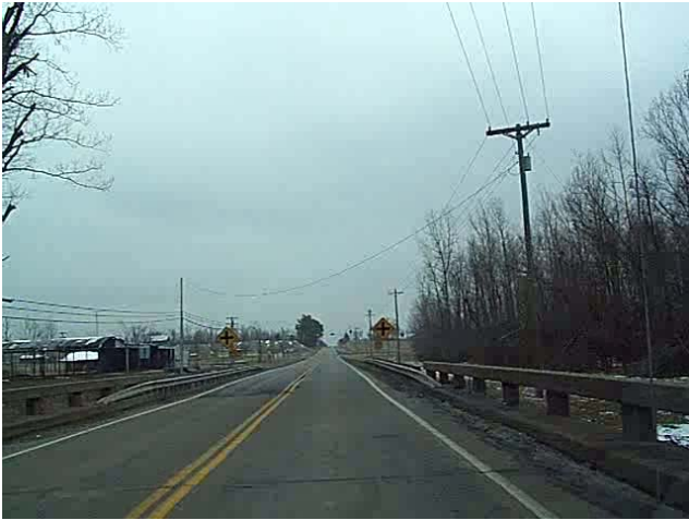
KY 54/Jack Hinton Rd Intersection
